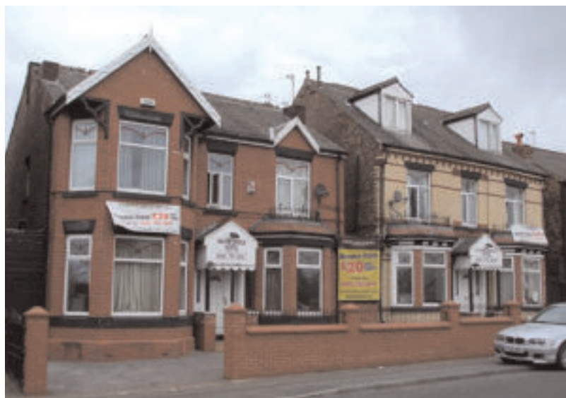
HOTEL BOSS ADMITS FIRE SAFETY BREACHES
